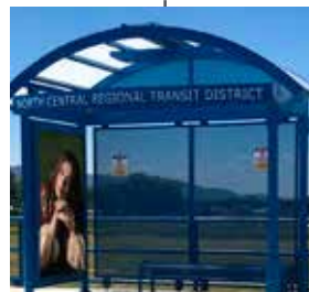
SIGNATURE PACIFIC ESPANOLA, NM Curved translucent roof and walls provide visibility beyond the shelter framing the beautiful surrounding landscape.
