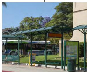
Four 17-ft spoke-style cantilever shelters offer flexible length adjustments to provide maximum shade. Amenities include steel strap benches, low-draw LED lighting, and back-to-back media display kiosks.
